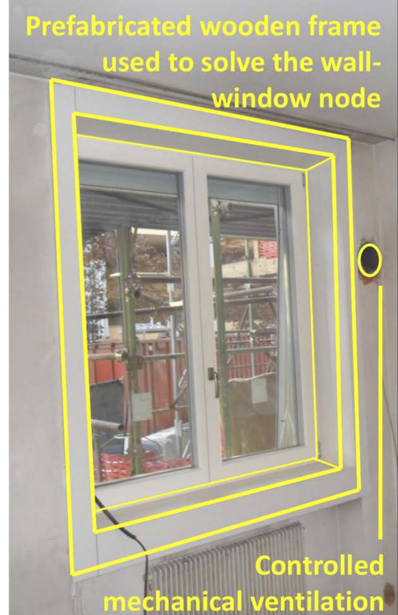
The new inserted window
