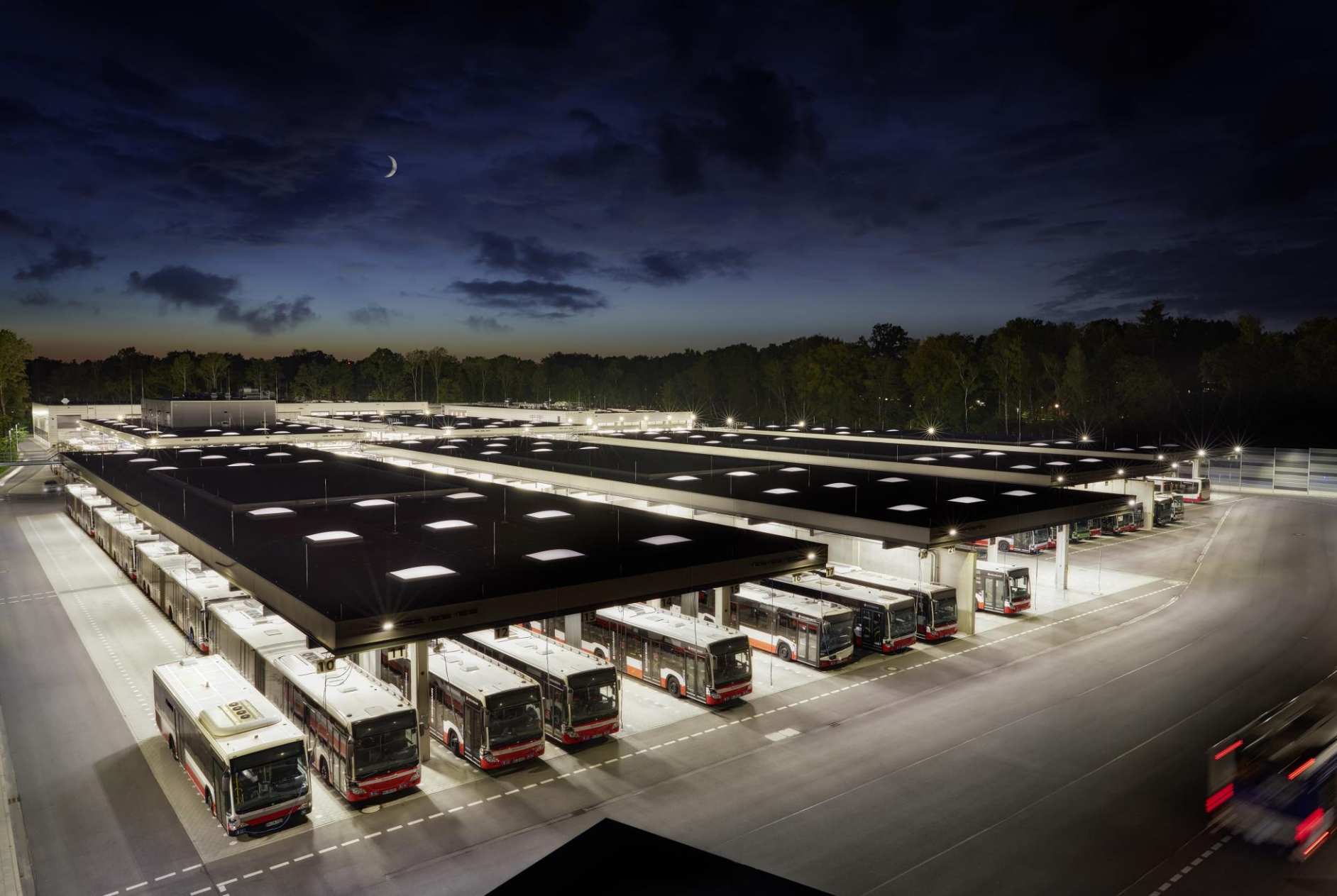
E-bus depot Hamburg-Alsterdorf | Source: Hochbahn
