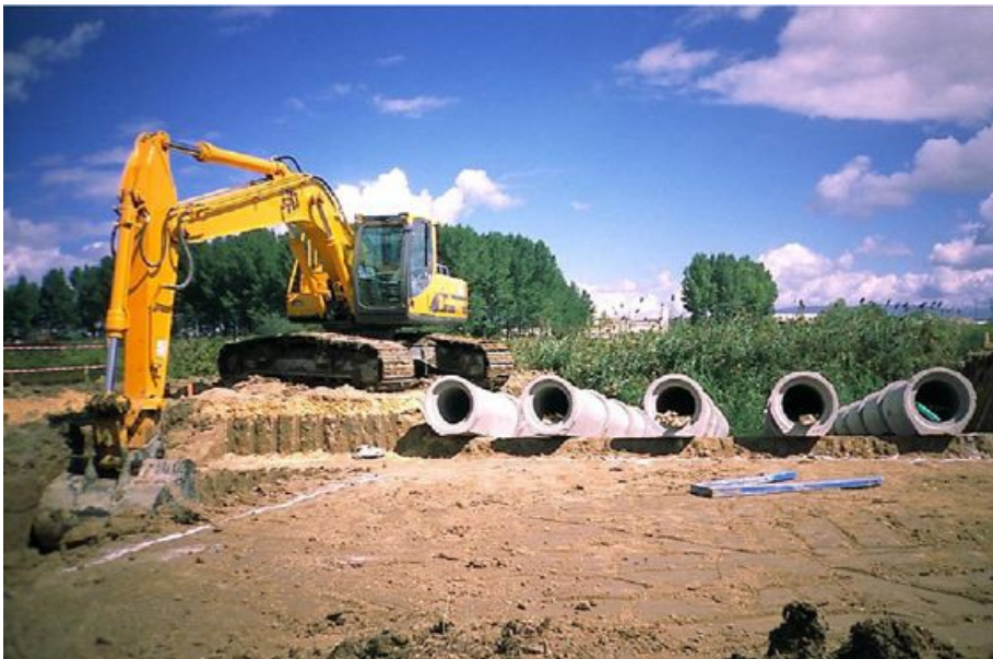
Restoration works in the Green Belt
