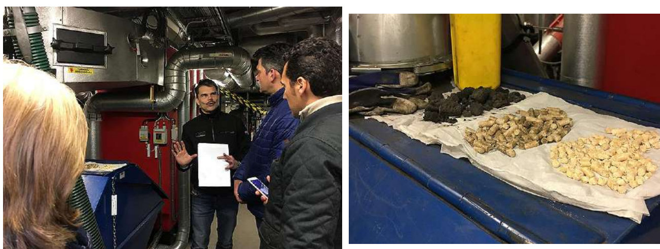
Figure 3. Images of study visit small scale district heating with biofuel.
