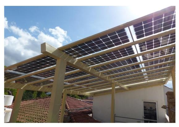
In the third installation 20 units of polycrystalline PV panels have been installed with a total power of 4,8KW covering a total area of 45 m2 of the skylight.
