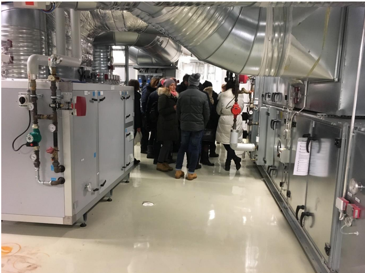
Visiting the Technical Room in the Alanurmo School.
