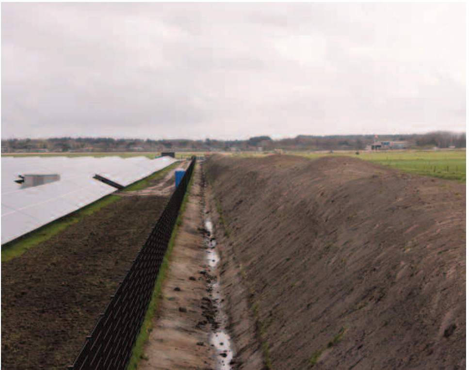
The new earthen wall that shields the Ameland Solar park. Photo Linde Egberts.
