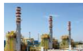
Figure 13 - Enipower power plant in Brindisi (Source: Enipower)
