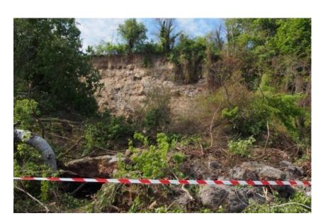
The erosional landside processes which should not be delayed, are on the slope of "Primorski park", on the First alley on the sea shore, over the 103 shoreline. The affected stretch is with length 80 to 50 meters and is located 300 meters from the slope of Alley First. The rocky slope is part of the Sea Garden and is state-owned.
