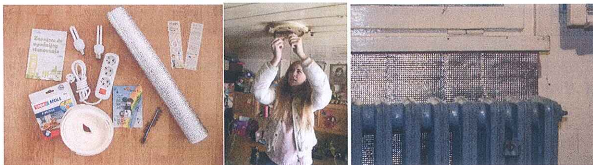
Figure 2 Example of the simple and low-cost EE kit provided to the visited households within the project REACH (left), energy advisor replacing an incandescent light bulb with LED bulb (center) and installed reflective foil (right)
