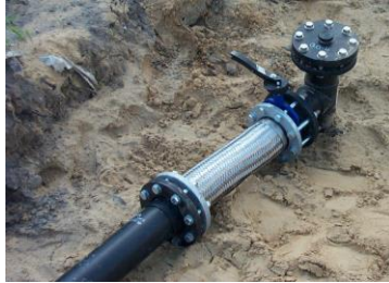
Gas wells for aeration and gas extraction
