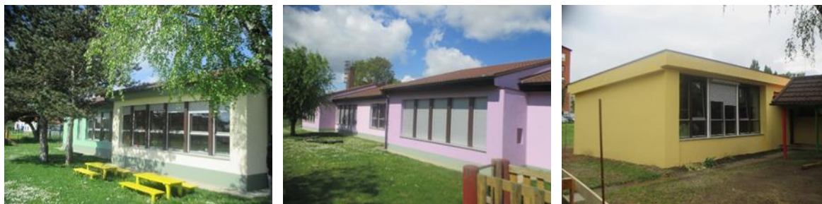
Figure 2: Energy renovation of Kindergarten Ptuj buildings.
