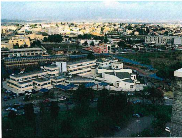
Brotzu Hospital, Cagliari, Italy
