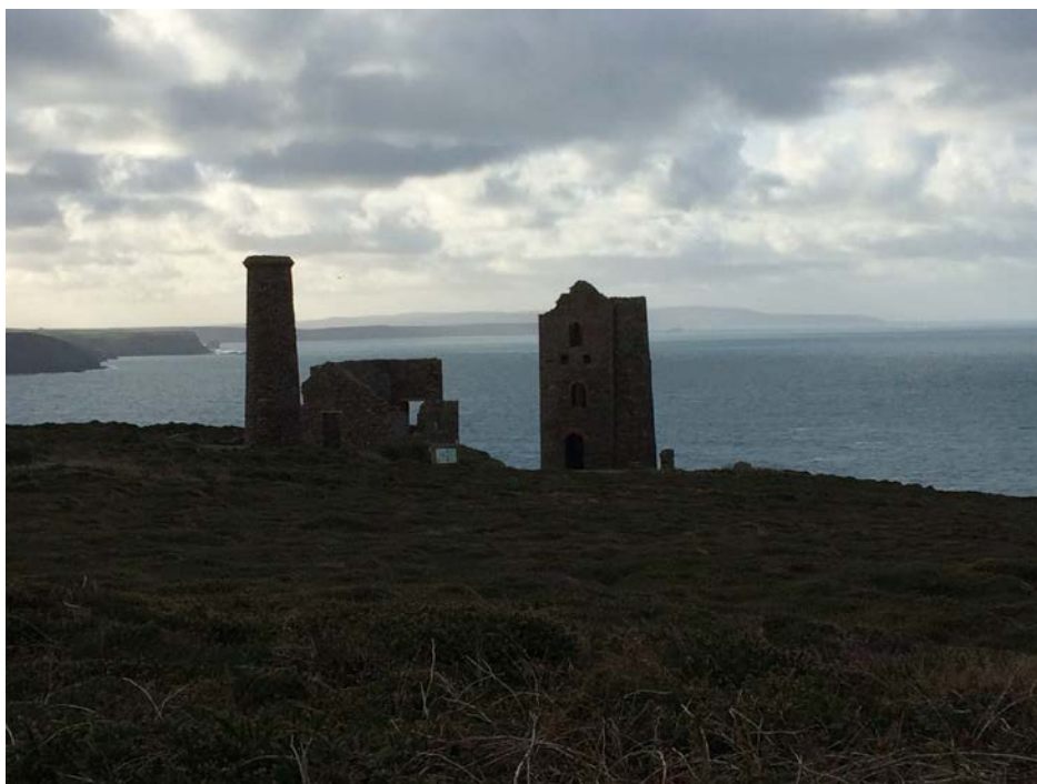
Figure 3: Wheal Coates engine house located near St Agnes in Cornwall's World Heritage Site.
