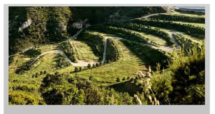
The restoration project is defined by a pattern of topographic configurations consisting of terraces, side slopes, a drainage system of internal fluids (separated from the external drainage network), a biogas extraction network, pathways and revegetation being conducted in phases.
