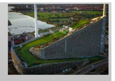
The new plant can convert 440.000 tons of waste into clean energy annually. It was designed by BIG as public infrastructure with a double function as tree-lined hiking trails and ski slopes were placed on its roof along with the tallest artificial climbing wall in the world on its facade. The ski slope is made of a specific plastic material like grass which is sprayed with an environmentally friendly oil to make it greasy or even snowy.
