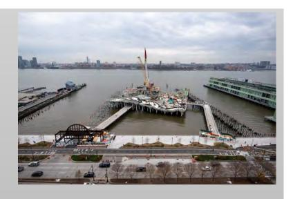
This urban park will stand on 132 tulip-shaped pillars that rise from the Hudson River. The concrete foundations will range from 15 feet to 62 feet in height, creating what the architects describe as "an undulating support structure" for the landscape, which is intended to resemble a leaf floating on water
