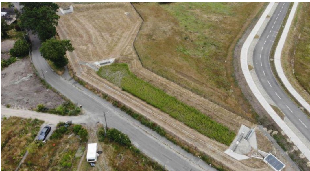
Fig. 3. The water treatment plant in Lurup - the pool is 66 meters long and 7 meters wide. The infiltration basin, planted with grass and reeds, has a volume of 1.6 million liters of water [32].
