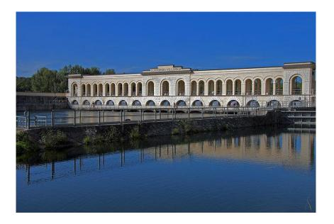
The dam allows to the Ticino river to be redirected towards two important canals: the **Industrial canal**, used for the production of electricity, and the **Villoresi canal**, used for irrigation purposes.
