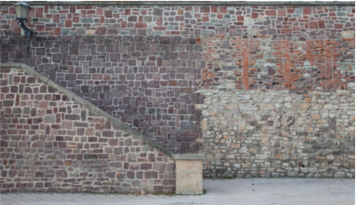
The *Fürstenwall* section of the city wall facing the Elbe river displays masonry from several different periods, and the mix of building materials creates the impression of a varied texture or calligraphic pattern
