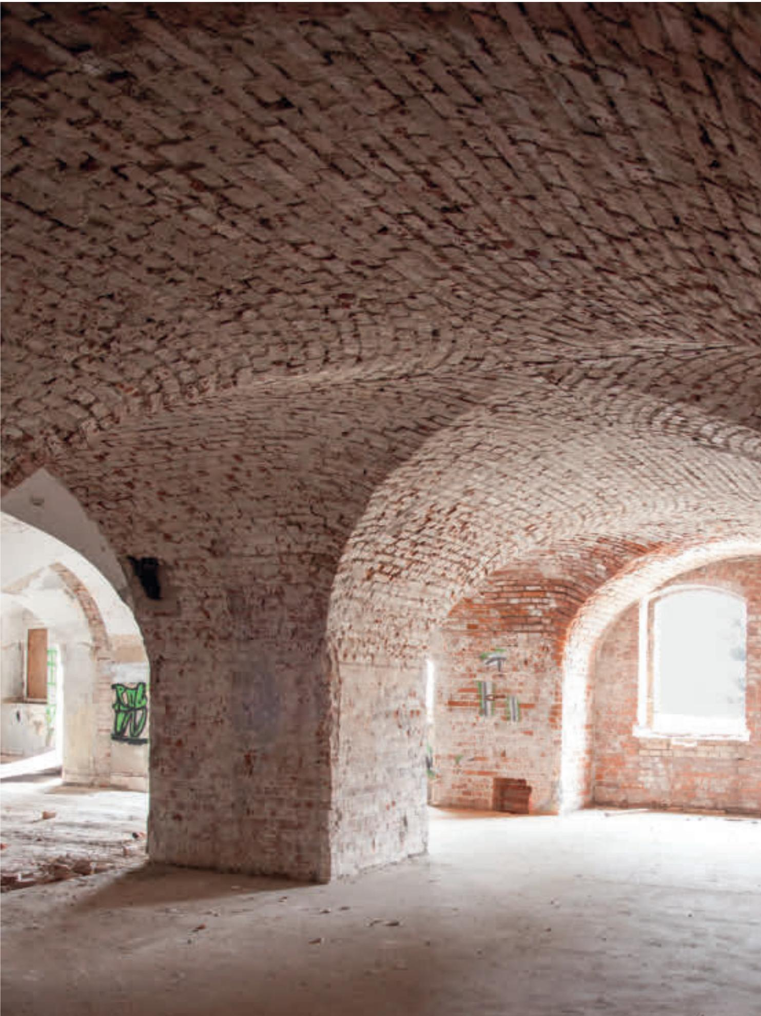
Massive pillars support the masonry vaults on the ground floor casemate of the barracks of *Kavalier Scharnhorst*
