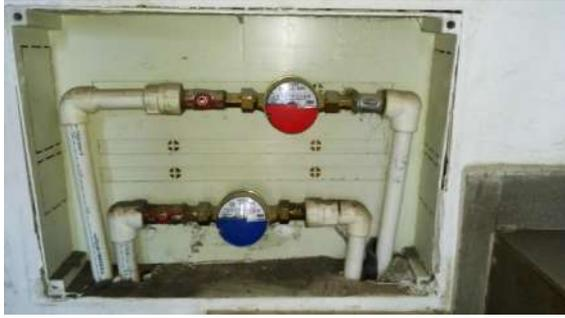
Fig.9. Cold and hot water meters
