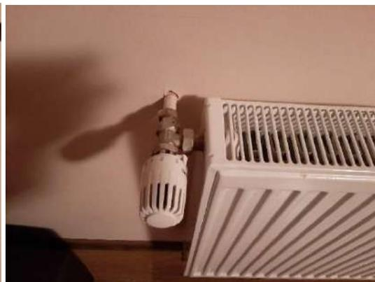
Fig.13. Radiator with mechanical thermostat
