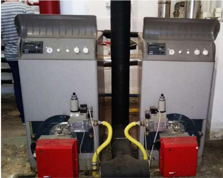
Fig. 6. Heating/ boiler systems for heating and hot water;
