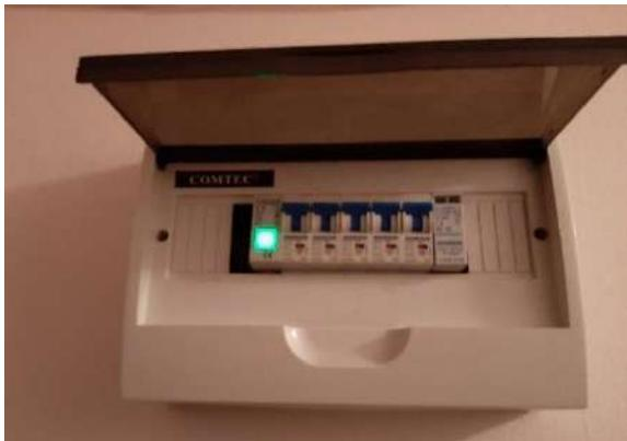
Fig.12. Electricity distribution panel with fuses
