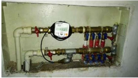
Fig.10. Heat meter with distribution pipes
