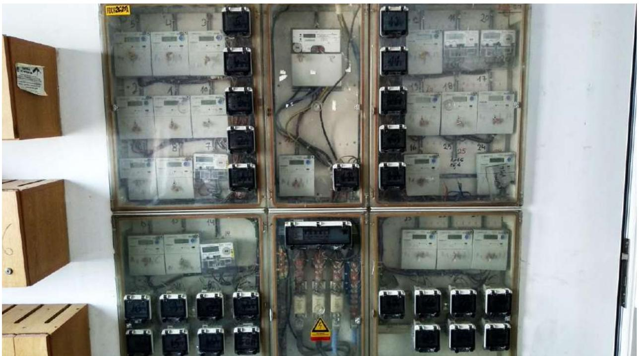
Fig. 8. General electric panel with fuses, protections, tri-phase general meter and individual meters (digital)
