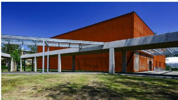
The metal-clad building has minimal windows because collections do not need light. The windows are oriented to the south only, where the museum staff have offices. The walls are built to absorb any higher humidity. On the other hand, when the building is dry, moisture will gradually be eliminated again.
