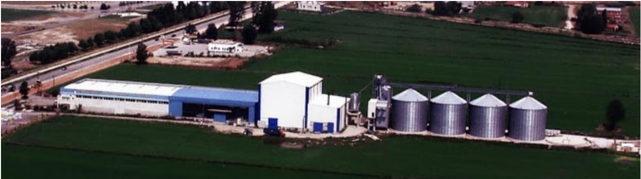
Figure 7 BEGAS AGRO SA industrial facilities (image free source from https://www.begasagro.gr )
