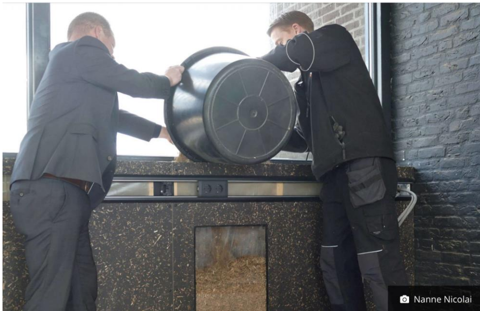
'Cigar plant' from the Better Wetter project insulates station building of Feanwâlden.
