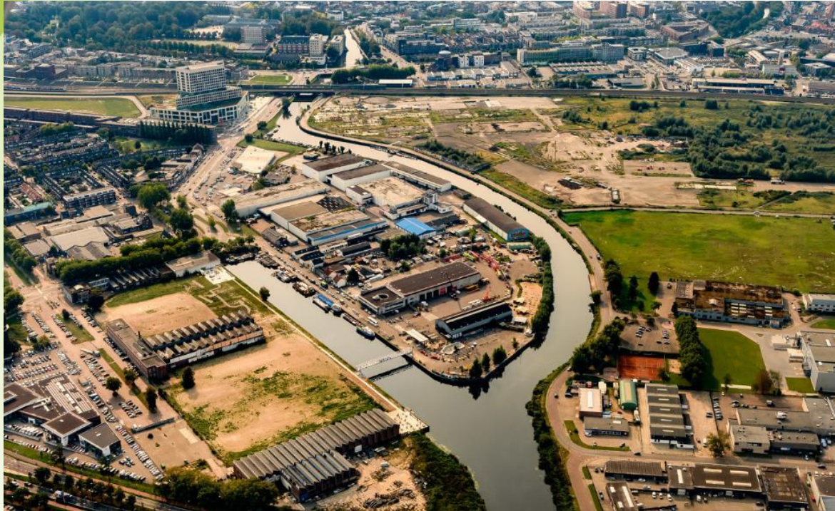
Overview over CrossMark area: "Strip" with halls, "Peninsula" (actual temporary use) and "Corbion"
